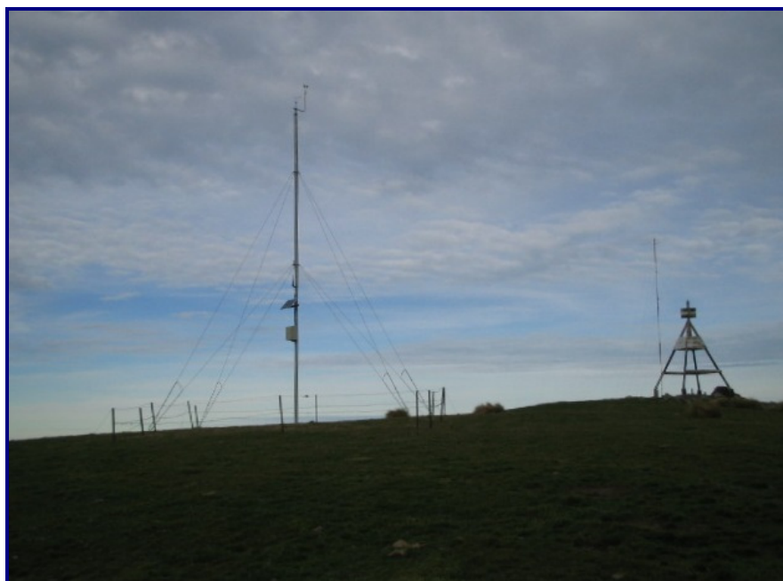
Mast Viewed from a Distance
