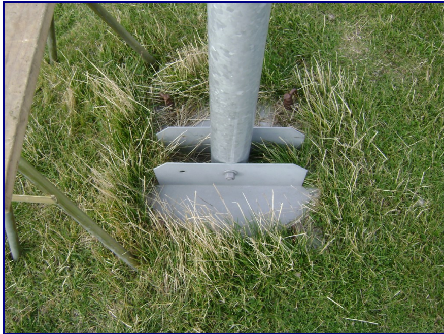
Mast Base Plate in Excellent Condition
